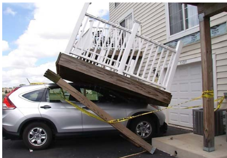
Photo: Deck with nailed-only ledger that was loaded by only father and daughter.
