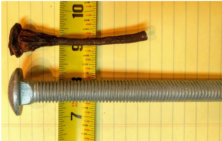
Photo: Comparison of a new 1/2-inch carriage bolt and a 1/2-inch carriage bolt after 13-years of coastal deck service
